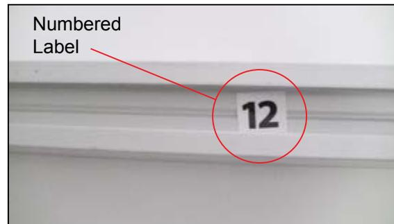
**Detail B:** Each extrusion contains a numbered label that corresponds to set-up instructions. The label is located within a groove of the extrusion (when possible). Visionary Design labels contain Black numbers unless otherwise specified.
